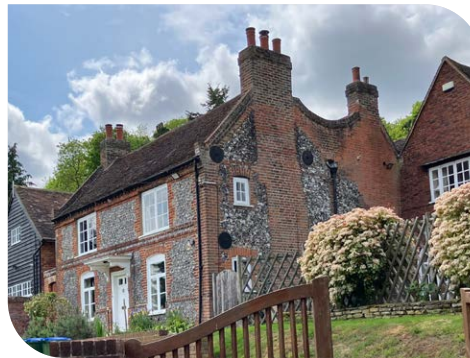
Tall brick chimneys
