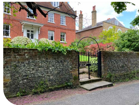
Knapped flint walls
