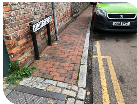
Red block paving from the late-twentieth century commonly found in the village
