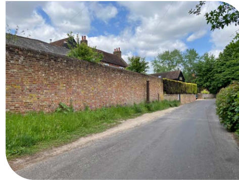
Red brick walls
